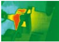
Motor: Bearing Problem
